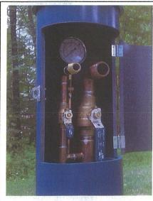
Optional attachment allows operators to super chlorinate and pressure test water main. After a five min component switch out, the operator is ready for samples.
